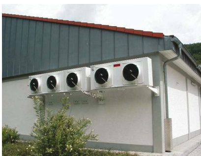
Small refrigeration units with ZIEHL-ABEGG Condenser with axial fans
