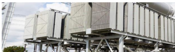
Transformatorcooling
