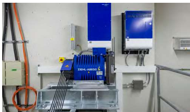
New - Gearless ZAtop drive with ZAdyn converter and ZAreC mains feedback unit Photo: BUTZ AUFZÜGE GmbH
